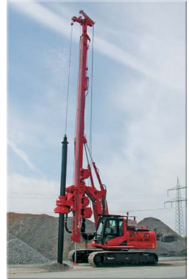
Depth measurement for sinking of foundation pillars with a rotary drilling system
